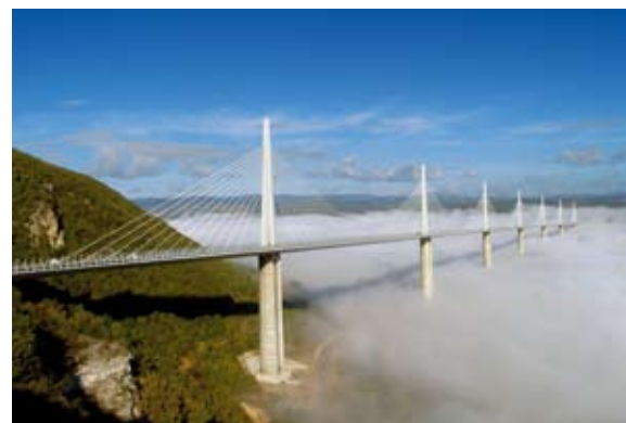
Fig. 32: Steel construction: Millau Bridge (France)
